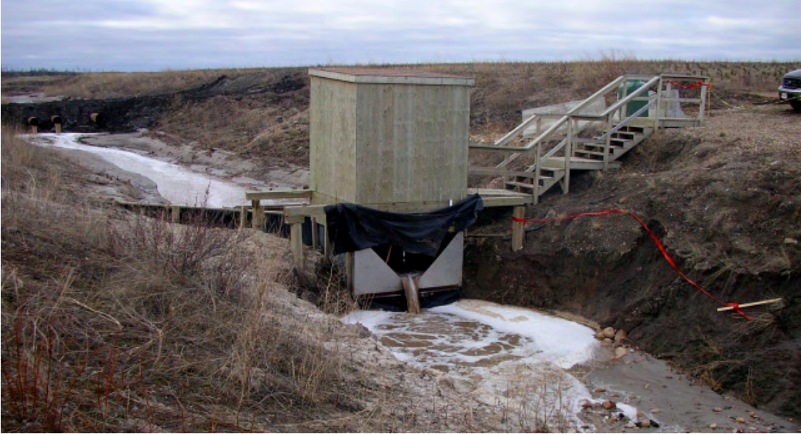
Figure 4.4 Photo of Syncrude V-notch weir during spring melt (photo provided by Syncrude).
