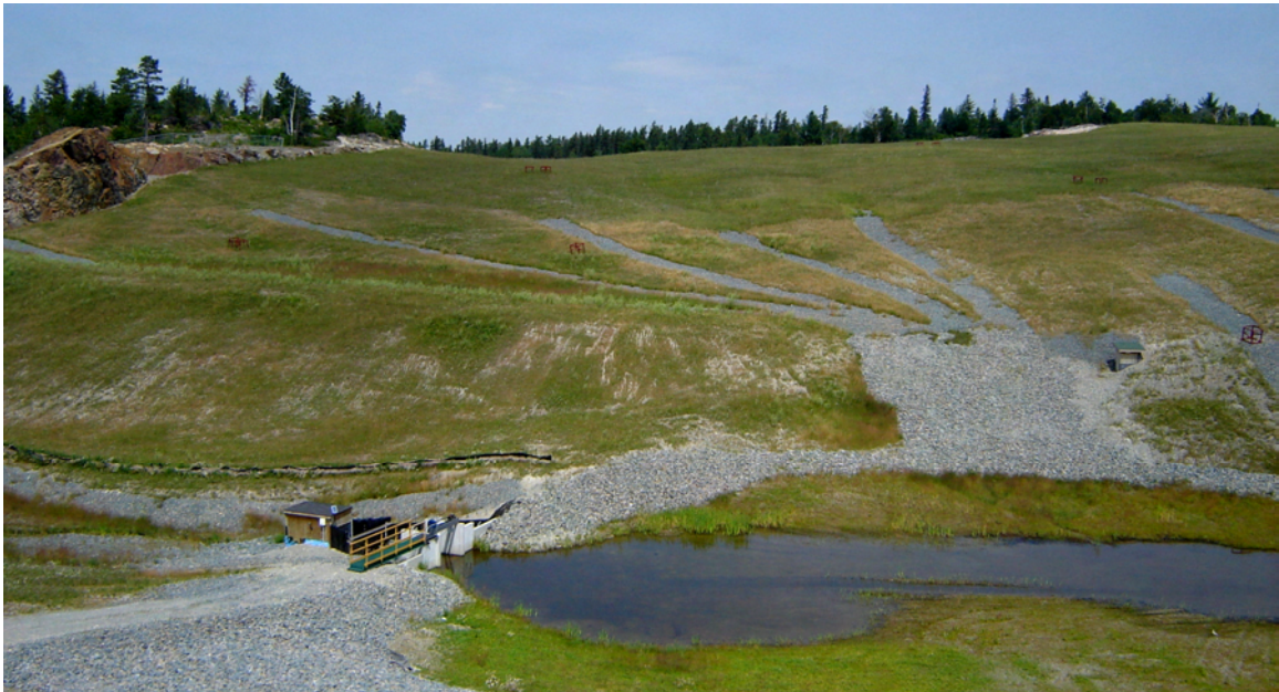
Figure 2.8 The Whistle Mine pit cover as of July 2007 (looking north) with the runoff collection and sedimentation ponds in the foreground.
