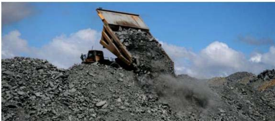
Figure 3-1: Conventional end-dumping MRS construction method.
